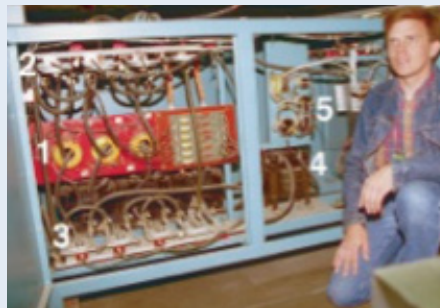
A typical high-power DC power supply
