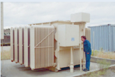
A 33,000 V, 10 A high-voltage power supply unit with radiators (left) and controls (front)
