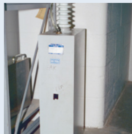
High-voltage capacitors, with shunting conductor (top)
