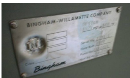
This N stamp nameplate is attached to the side of the EDP pump.
