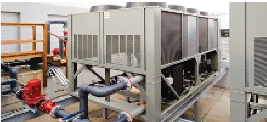
Air-cooled chillers installed outdoors.
