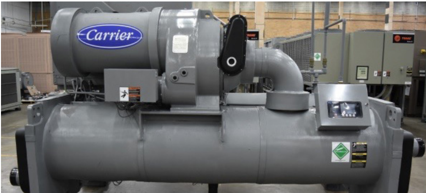
Indoor water-cooled chiller (205 ton).
